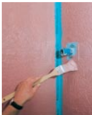
4. Place PCI-waterproofing gasket (wall) over the pipe connection protruding from the wall and cover with PCI-Lastogum (red).
