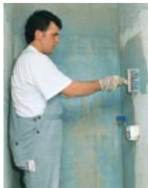
1. Priming: Prime absorptive mineral or gypsum-based substrates and plaster boards with PCI-Primer g.
