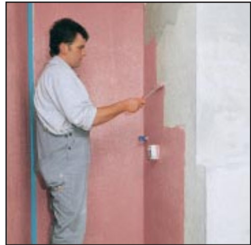
Application of undiluted PCI-Lastogum to the substrate by roller, brush or trowel.
