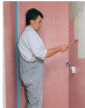
2. Apply undiluted PCI-Lastogum (red) to the substrate as a first protective coating to cover its entire surface.
